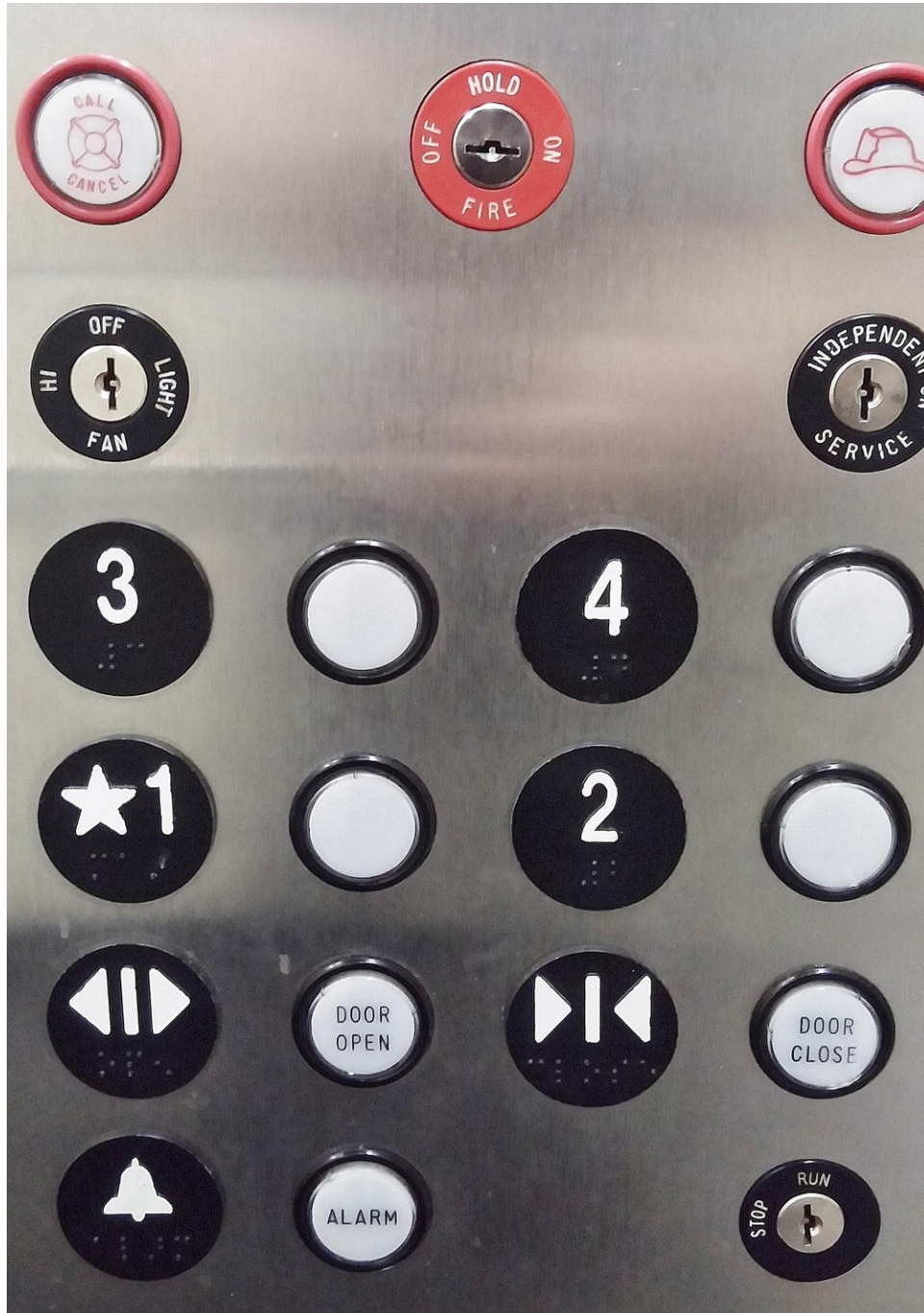
Figure 18-2. Elevator “door close” buttons are often false buttons that have no effect on the door’s operation 4
